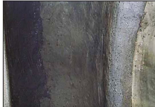
ARC BX2* and ARC 855 applied to pump volute
